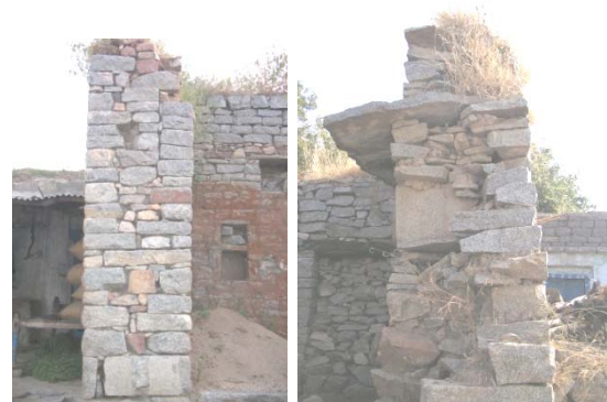
Fig. 6: Ashlars & Rubble wall construction
